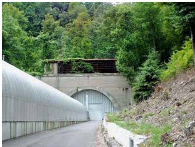
The Laurel Hill Tunnel in Pennsylvania
